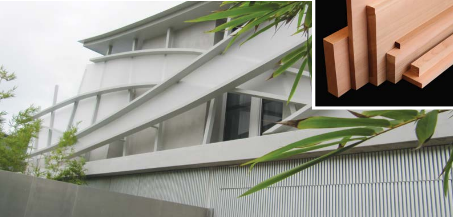
Curved cedar screen sections – laminated DAR
