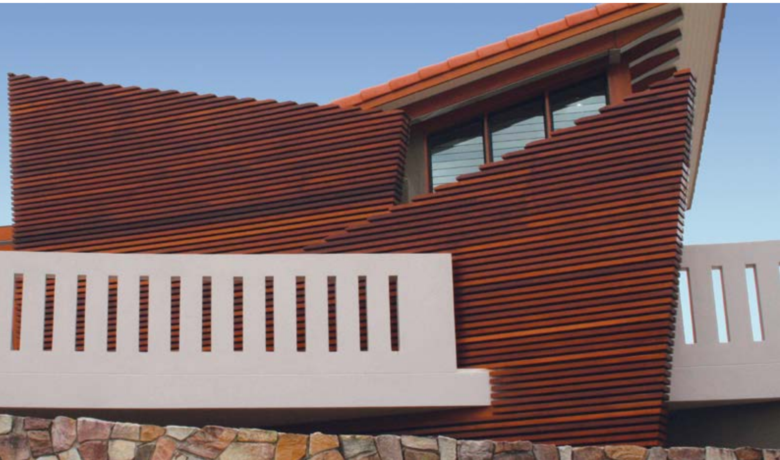
Architectural screen — square dressed sections
