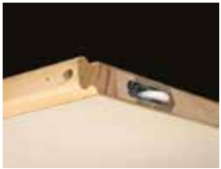
WHEEL ASSEMBLY Also pictured is timber finger grip on door edge
